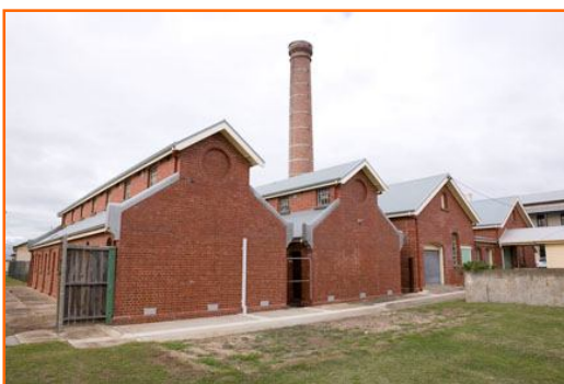
Bath block & disinfecting building and boiler house
