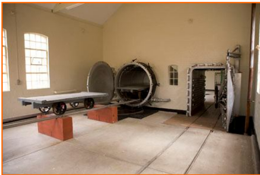
Interior of disinfecting building and boiler house
